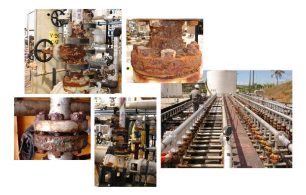
FIGURE 1 – Examples of Flange corrosion
